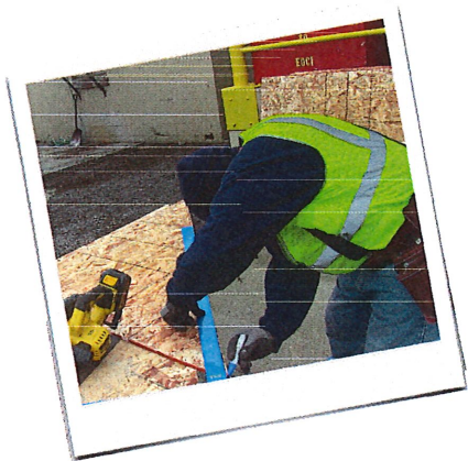
Benjamin Edwards cuts out ply board to be used on the roof repair project.
