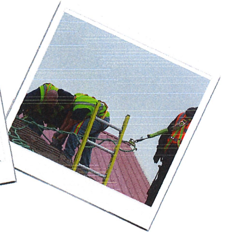
Trevor Sorensen and Pablo Perez repairing the recycling shop roof.
