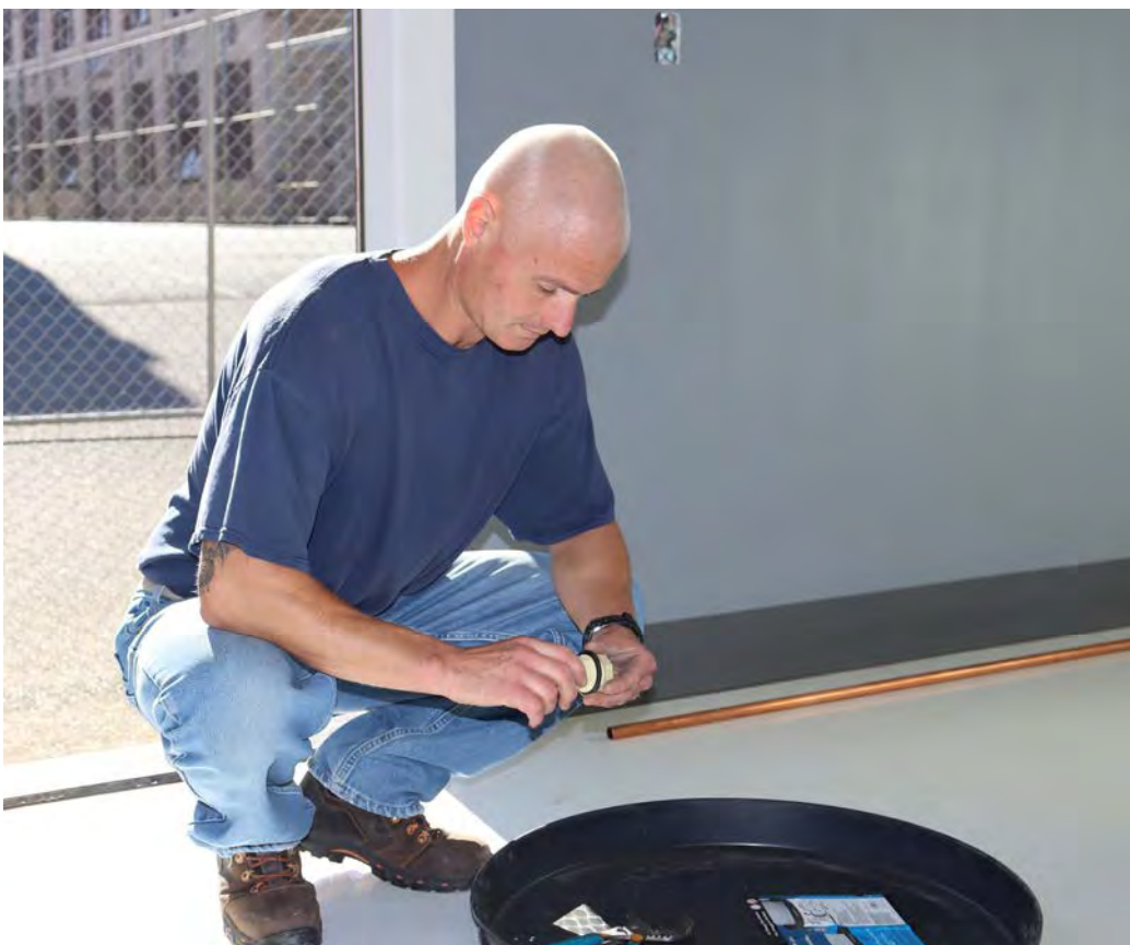
Hardegger preps water heater parts for Westgate.
